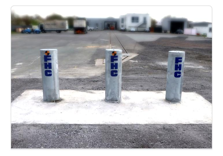
The FHCM50 Fixed Shallow Mount Bollard was designed to protect the perimeter of the protected area. Offers maximum security against unauthorized wheeled vehicles while enabling unhindered pedestrian access. These robust bollards are crash-tested to internationally accepted standards and feature shallow foundations for easy installation.
